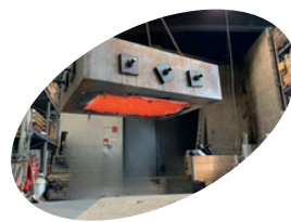
Passive Fire Protection
